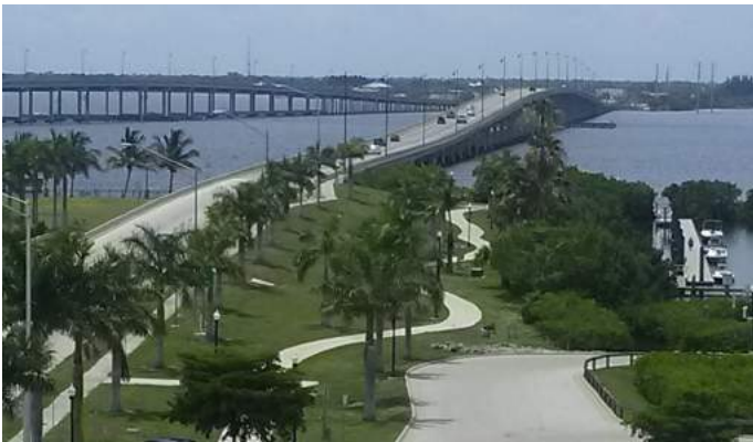
US 41 Bridge over Charlotte Harbor
